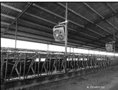
Fig. 2: Fans placed so that they cool cows at the bunk; moving air over wet animals removes more heat than when they are dry and means we need less soaking overall.
