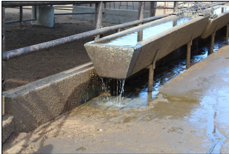
Overflowing troughs waste water that could be utilized elsewhere.
